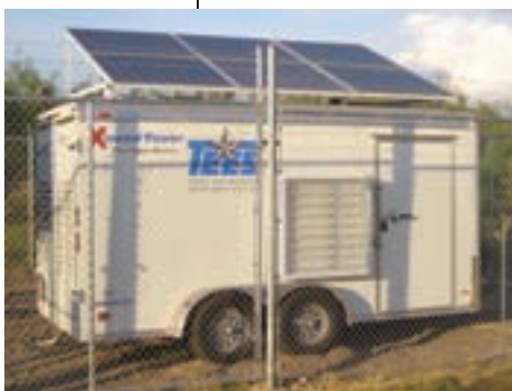
SECO brings electricity to La Presa residents.
