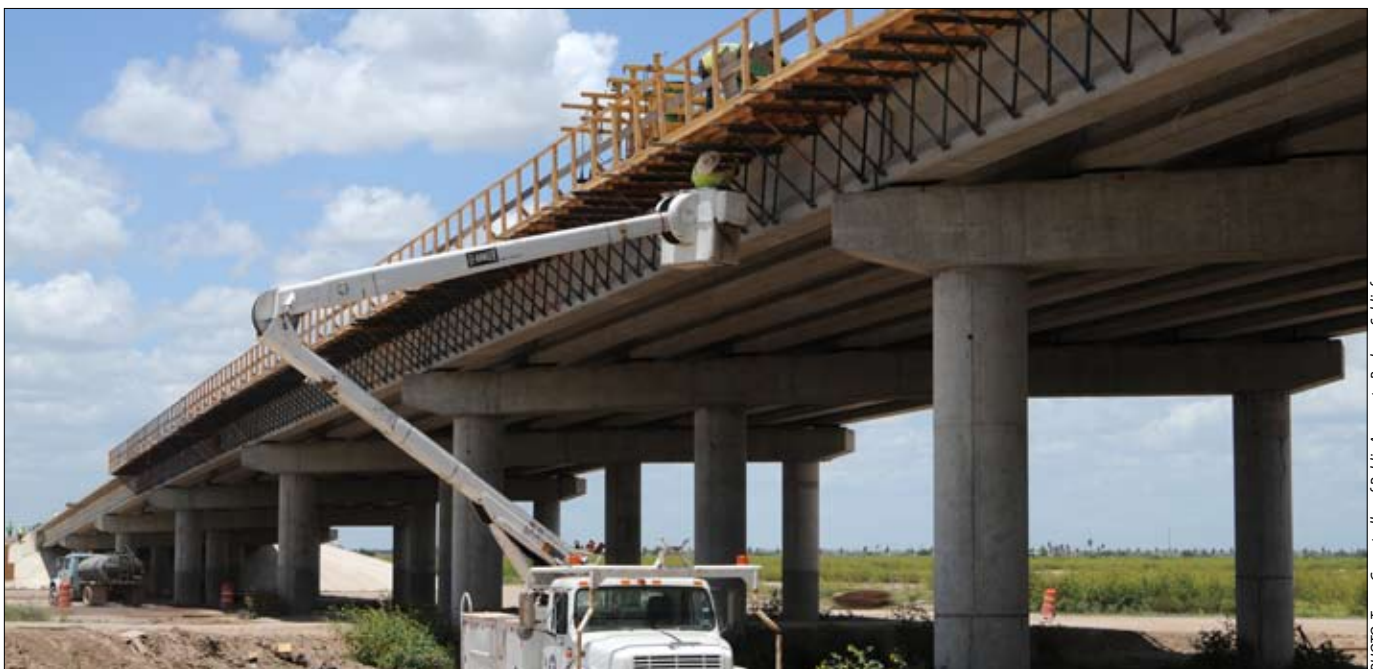
Anzalduas Bridge Construction, McAllen, Texas
