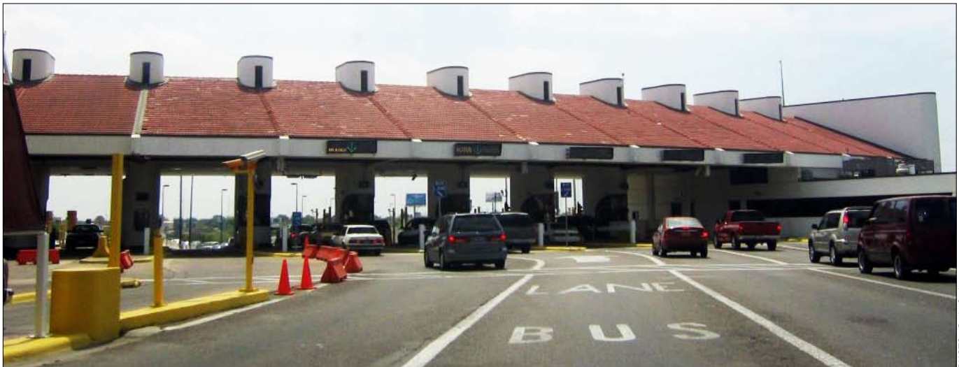
International Bridge Toll Booth, Laredo, Texas
