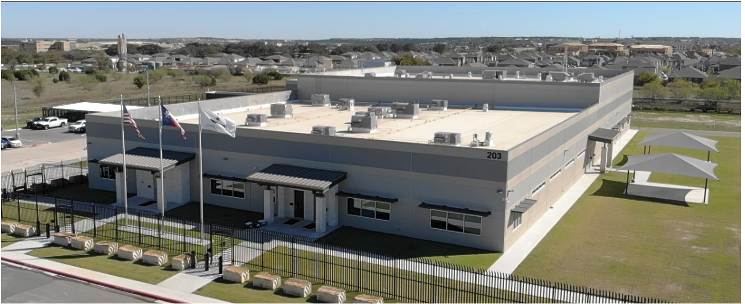
Texas Bullion Depository in Leander, Texas
